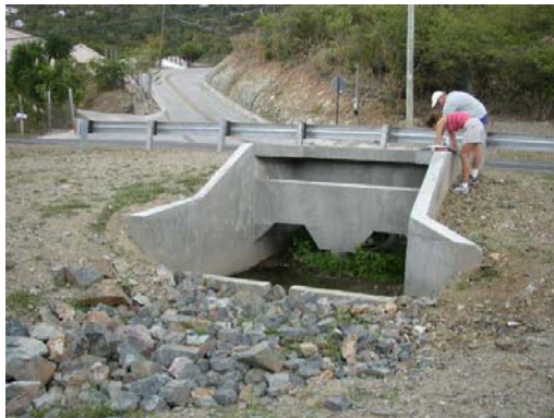
Figure 5 – Energy Dissipation Structure
