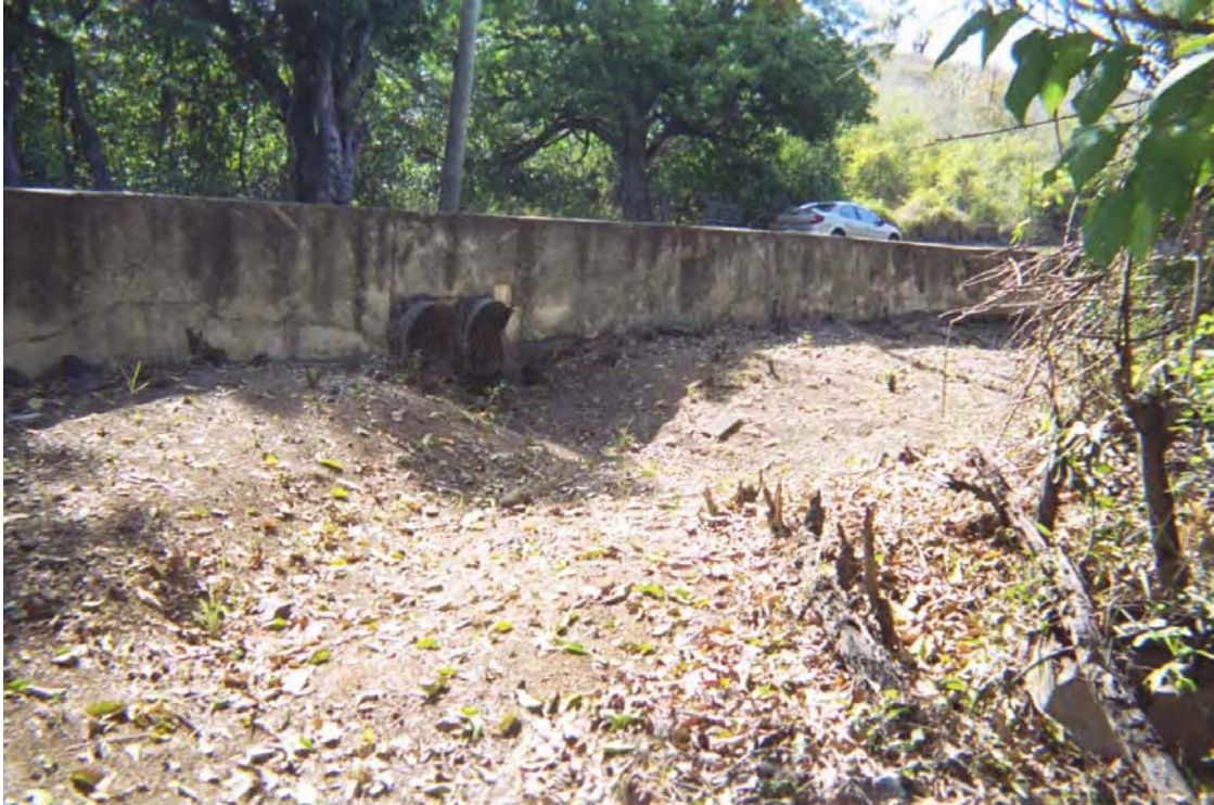
Photo 7: Eastern (Downslope) Side of Culvert along Smith Bay Main Road
