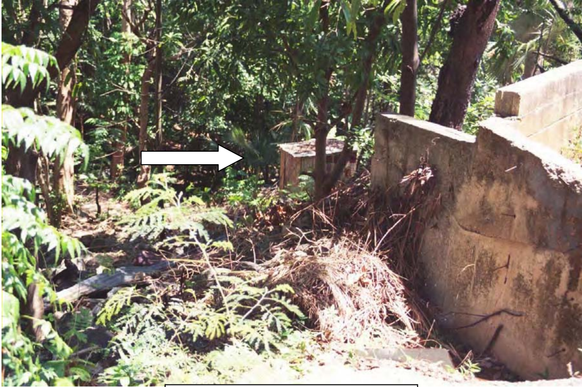
Photo 26: Building in Contant Gut
