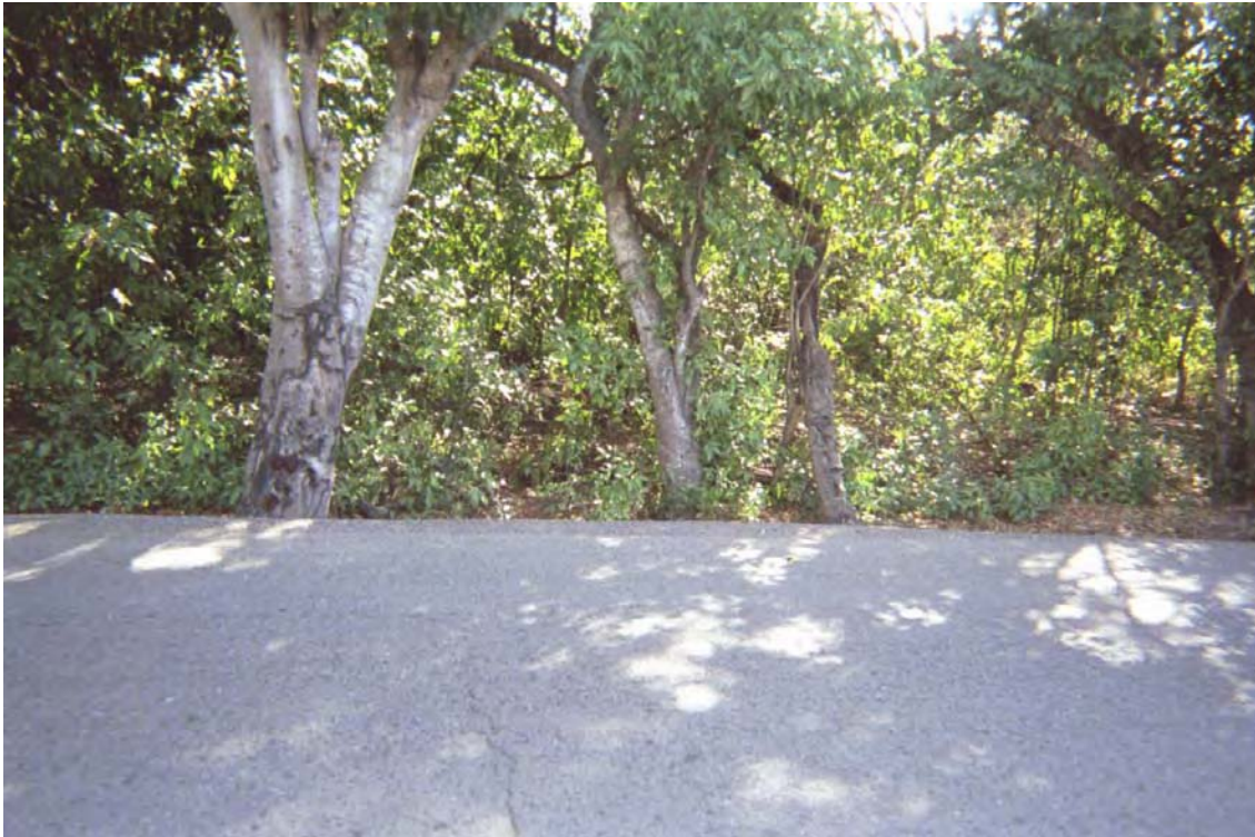
Photo 6: Western (Upslope) Side of Culvert along Smith Bay Main Road
