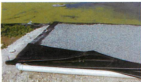
Figure 1. Earthen pad with EPDM liner and gravel for the geotextile bag.
